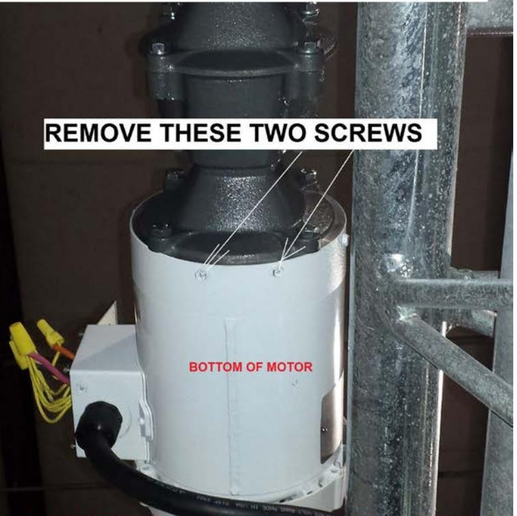
**NOTE: THIS BULLETIN APPLYS TO ALL LANDA MOBILE SYSTEMS PORTABLE TOWERS USING A LEESON BRAND ELECTRIC MOTOR IN THE LIFT WINCH ONLY. NO OTHER MOTORS, TILT NOR HYDRAULIC PUMP, ARE EFFECTED BY THIS PROCEDURE. IT'S PRECAUTIONARY ONLY TO DRAIN ANY ACCUMULATING MOISTURE IN THE MOTOR**
